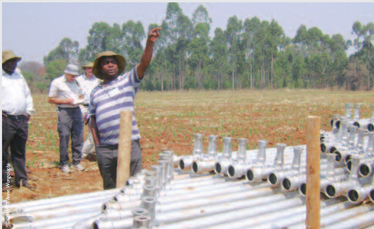
Maize breeder, discussing irrigation pipes to be installed at the Chiredzi Research Station in Zimbabwe.
