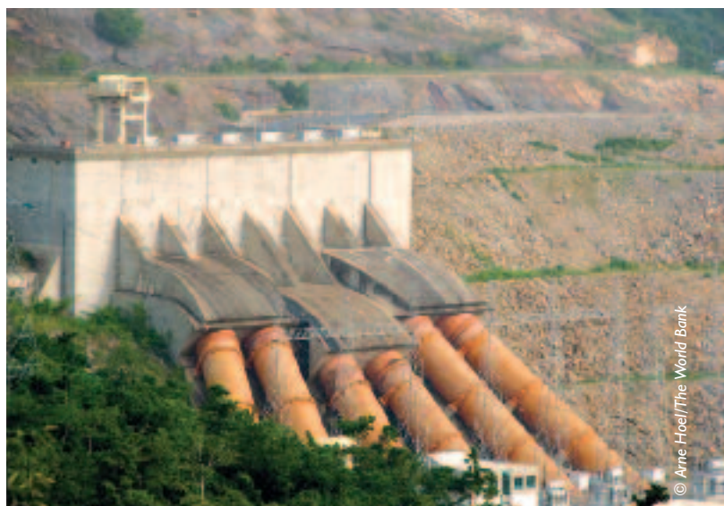
Hydropower plant in Ghana.
