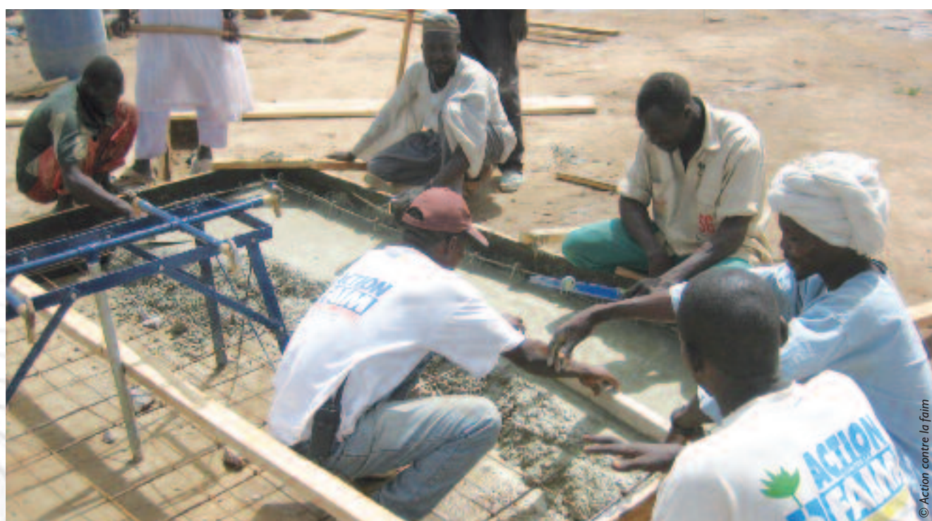
Building a water point, Chad.
