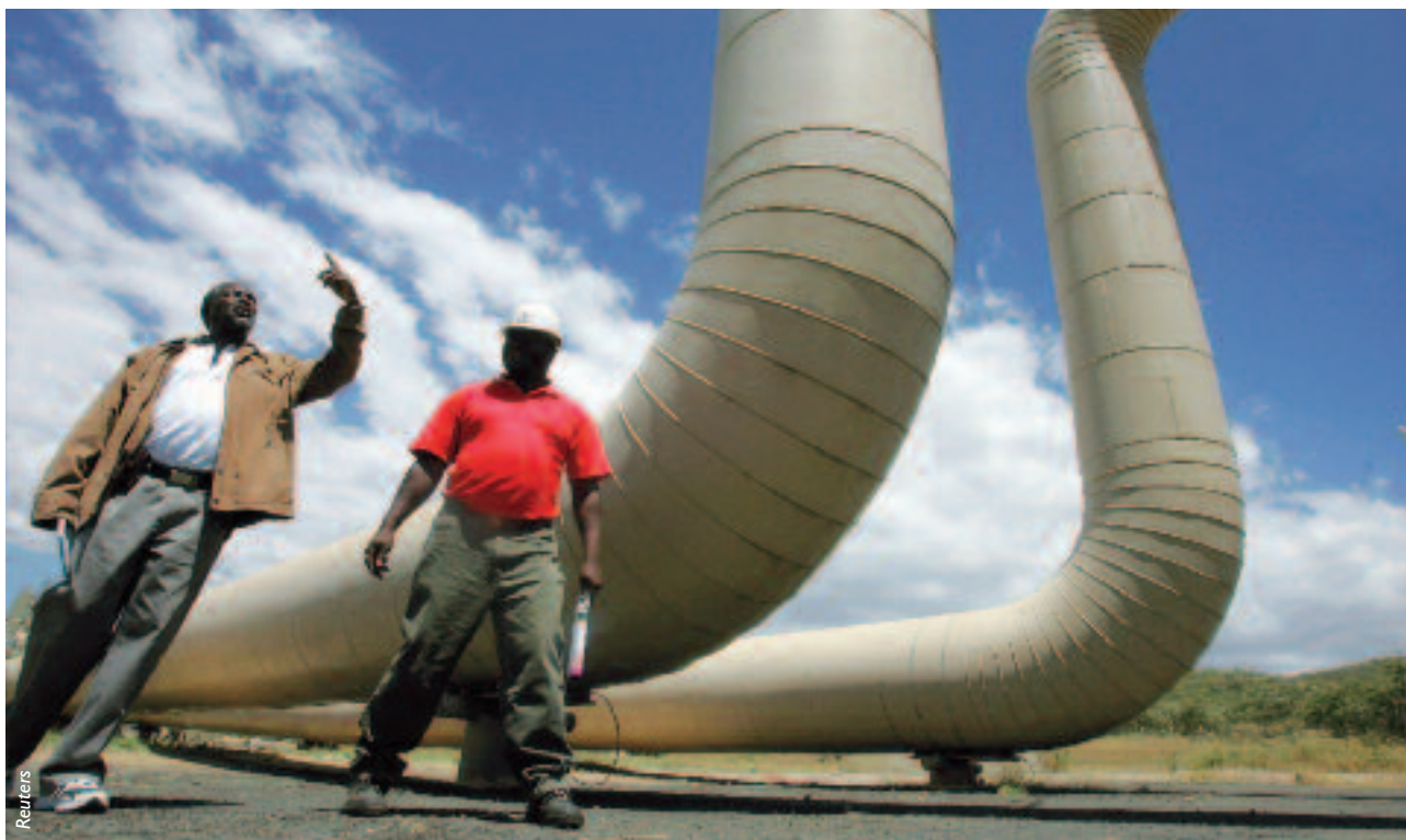
Geologists at the Olkaria Geothermal Energy Power station in Naivasha, Kenya.
